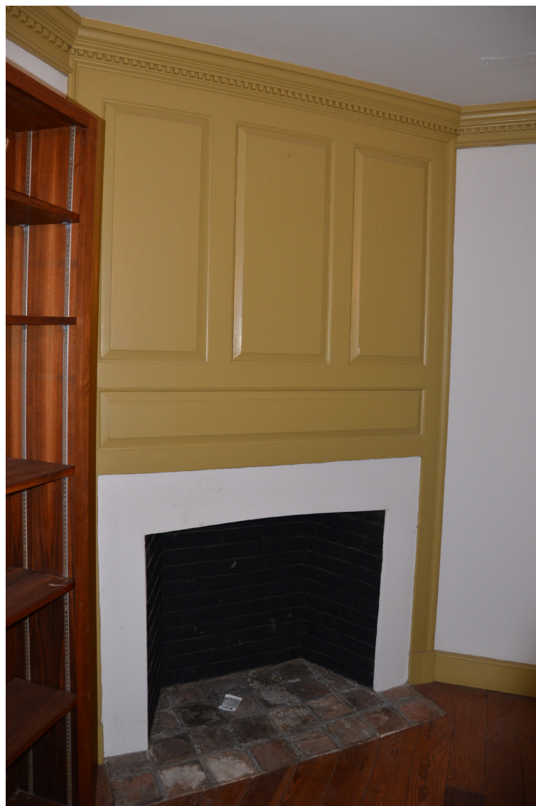
Fireplace panel and overmantel
